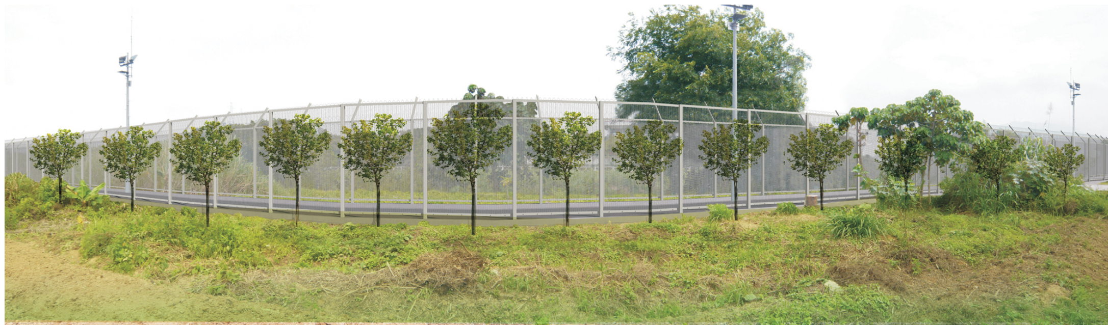
View displaying the 3D Model of the Project with Mitigation at Day 1 Operation
