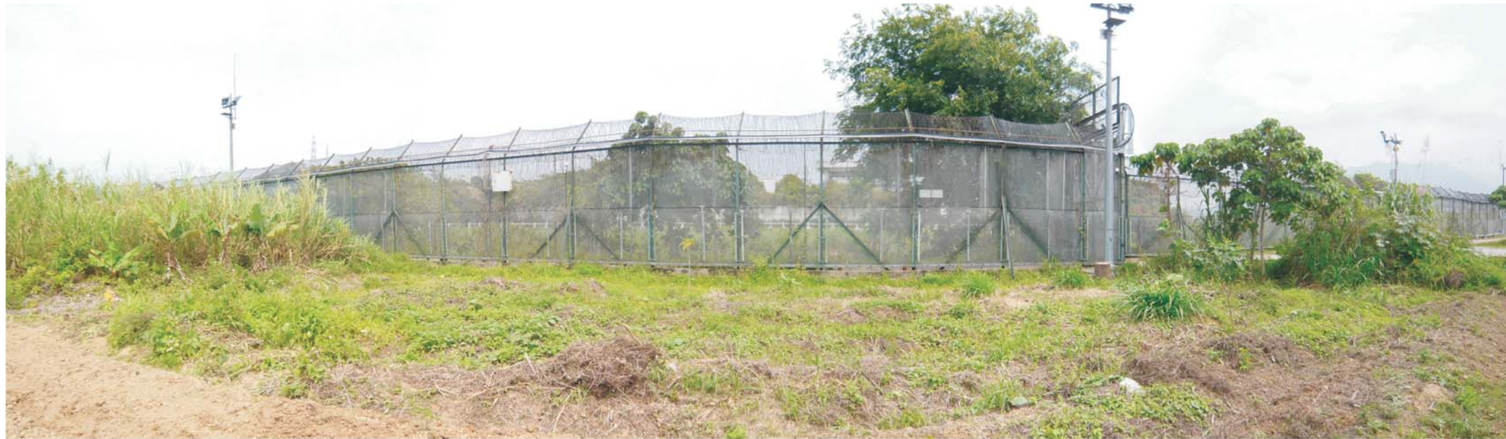
Existing view from Ta Kwu Ling Village Towards the Project Site
